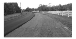
Cracked and broken pavement was ground up on Talbert Hill and Codfish Hill and prepared for paving in 2015.
