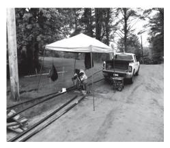
year old badly corroded 1 <sup>1</sup>/<sub>2</sub>" galvanized pipe with a brand new 2" HDPE and installed a new 2" automatic blow off hydrant at the end of the line. In our second spur we replaced an undersized 3/4" plastic service line that ran out 500 feet and serviced 5 homes. We tapped into the main line and installed a new 2" HDPE pipe along with new curb stops and new curb
